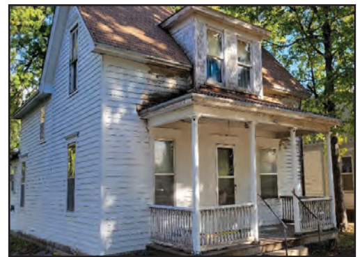
The house after some primer is added.
